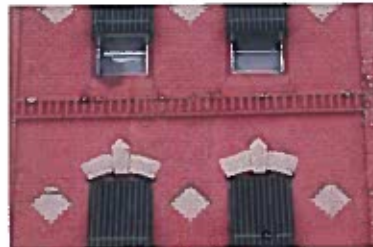
Elaborate brick detailing should be preserved.
