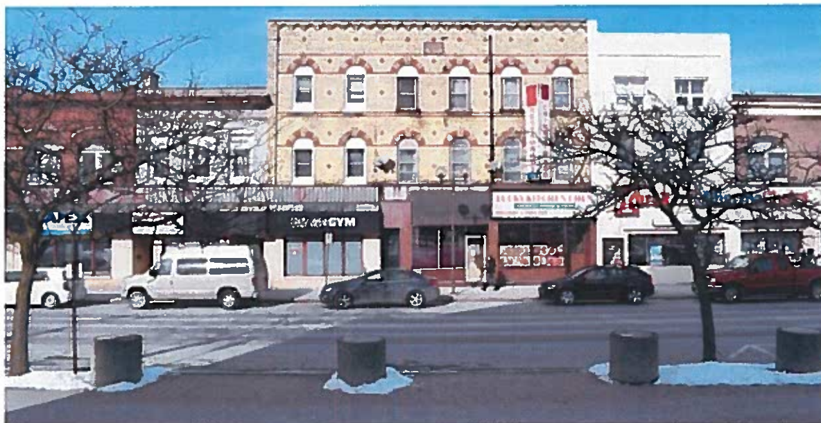
Plate 1: Typical building form of the Talbot Street Streetscape.
