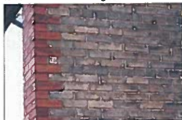
Brick may differ on front and side elevations. This was common for historic buildings and should be maintained.
